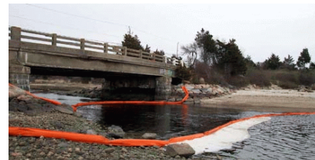
Figure 3-3: Boom deployed at Route 54 bridge crossing.
